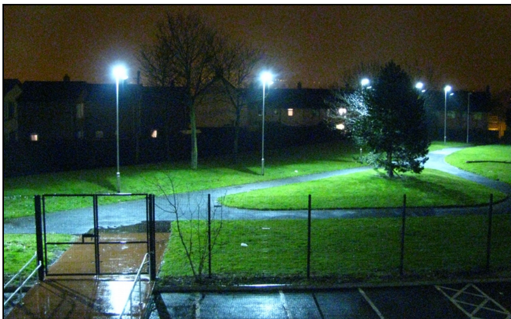
New lighting for Suffolk side of SRRP estate
